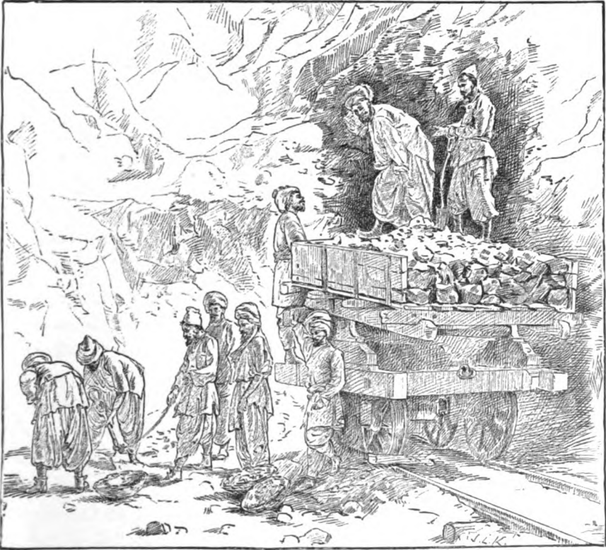
To Kandahār "—Tunnelling for the Railway through the Khojak.
